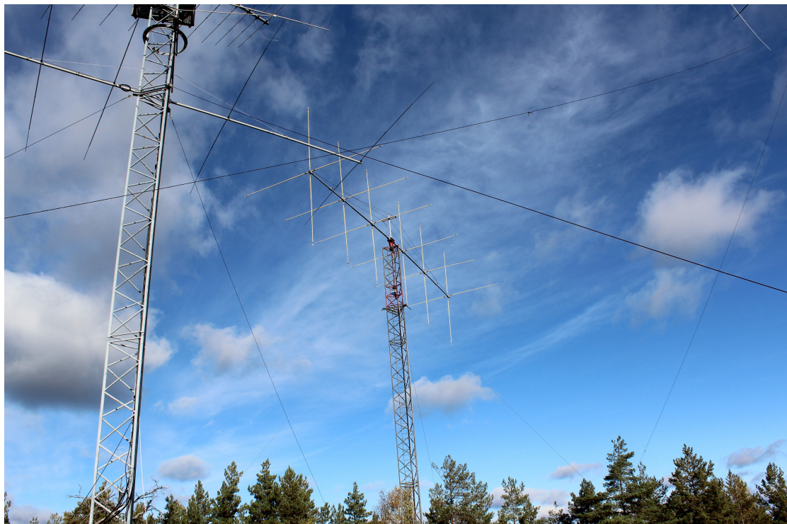
Antenna farm at Mill Hill (sk0ux.se)
