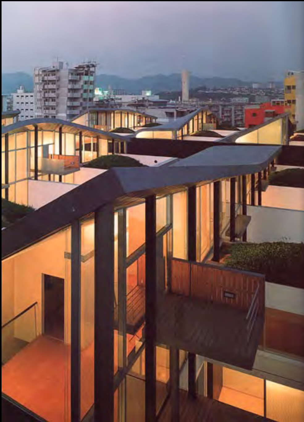
Nexus World Fukooka, NL, 1991 - View over roofscape
