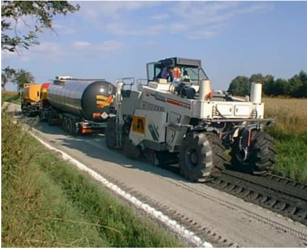
FDR WITH FOAMED ASPHALT
