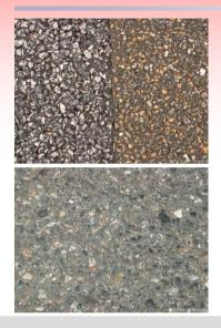
Description: Areas of HMA pavement where the portion of aggregate extending above the asphalt binder is either very small or there are no rough or angular aggregate particles.
