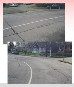
**Description:** Cracks in a flexible overlay of a rigid pavement. The cracks occur directly over the underlying rigid pavement joints. Joint reflection cracking does not include reflection cracks that occur away from an underlying joint or from any other type of base (e.g., cement or lime stabilized).
