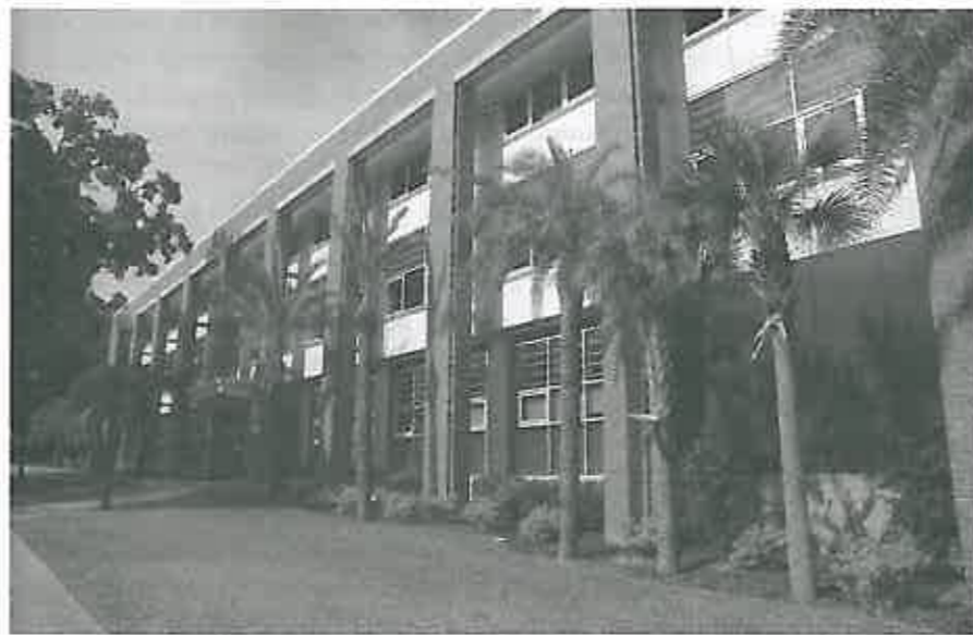
FIGURE 7.1 Rinker Hall is a high-performance LEED-certified Gold building at the University of Florida that incorporates advanced energy strategies. (Photograph: Michele R. Moretti.)
