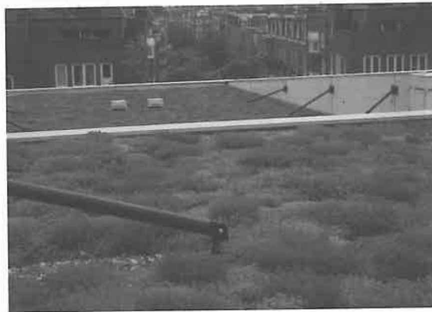
Greenroofs or eco-roofs are now common in Europe, especially in Germany, Austria, and the Netherlands. Shown here is a multilevel greenroof at the GWL-terrein housing complex in Amsterdam.
