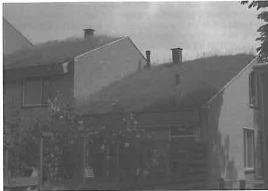
Greenroofs are also beneficial in more suburban settings, such as in the Romolenpolder neighborhood in Haarlem, the Netherlands.
