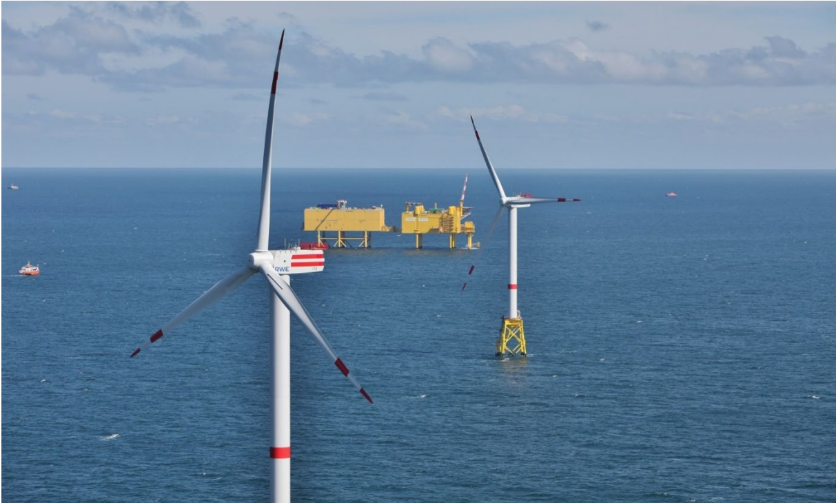
Picture of an offshore HVDC station (source: PROMOTioN/TenneT)
