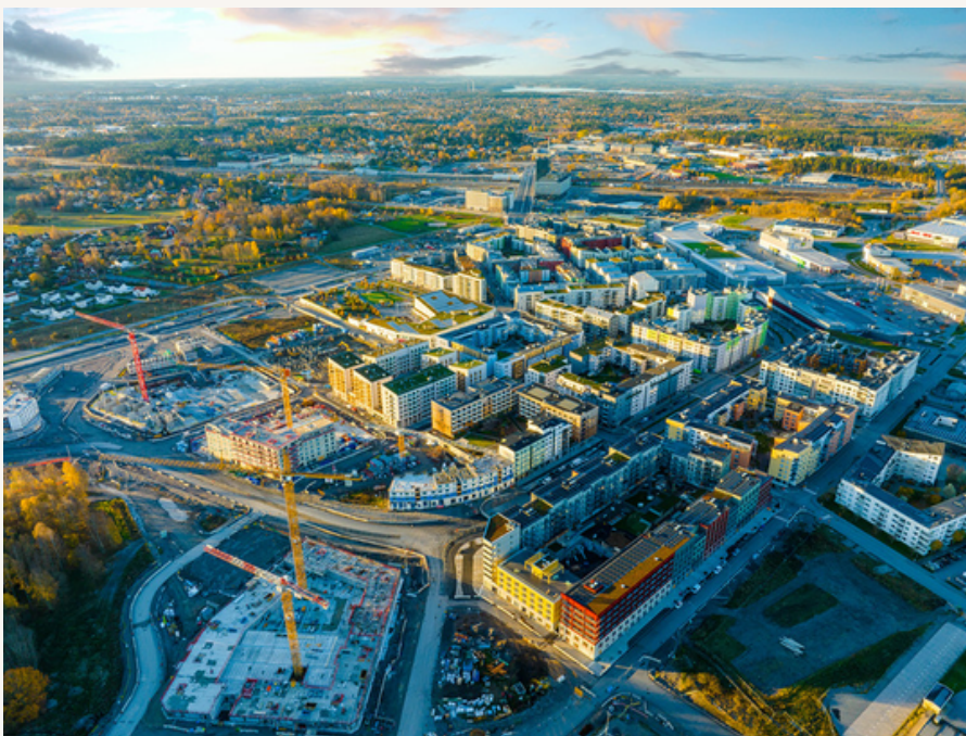
Foto: Construction of Barkabystaden, one of the main current urban developments of the municipality. Source: Järfälla kommun
