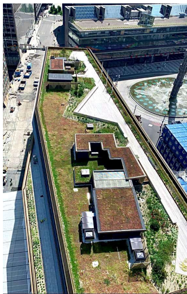
Figure 8: The roof of Sergelhuset located in the heart of Stockholm, fitted with Urban Green own Sedum roof (Urban Green A. n.d. Accessed 27 Nov. 2023)
