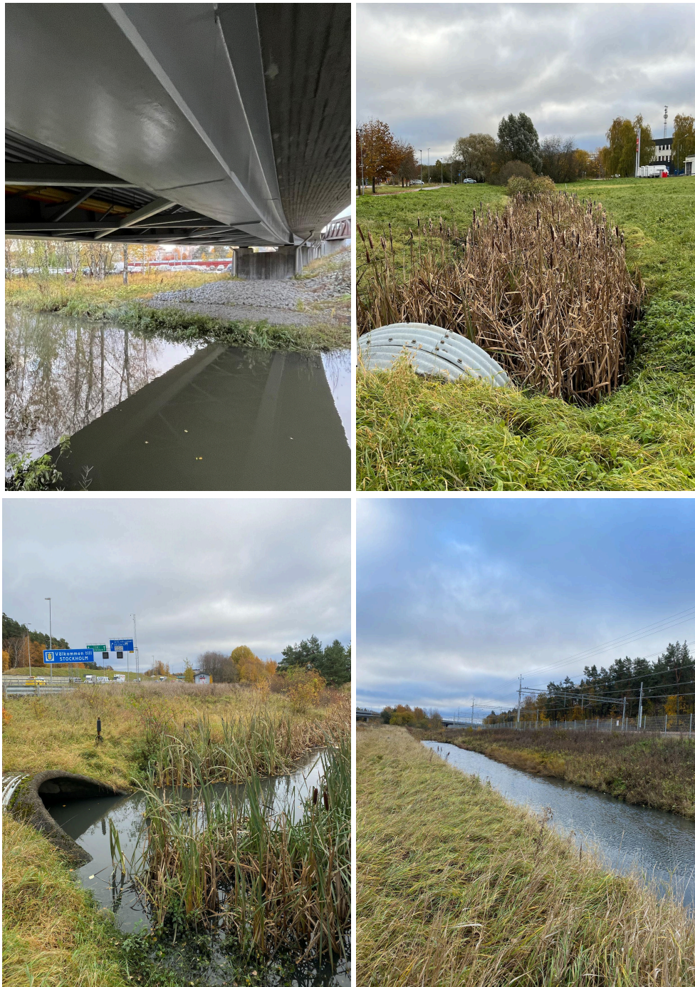
Figure 5. Images from site visit on 2023-11-01 (By authors)
