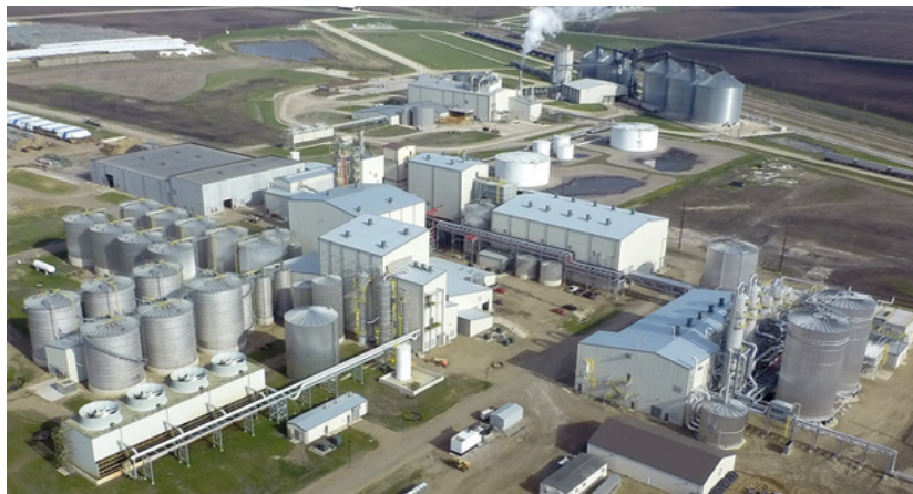
Fig.1. Poet-DSM Project Liberty is a cellulosic ethanol plant that uses engineered yeast strains, together with many other technological advances, to produce renewable biofuel from corncobs, leaves, husk and some stalks. Image: dsm.com
