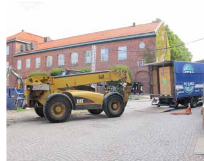
Above: Each compute rack arrives packed in a crate. Here one of the crates is lifted from the delivery truck with a forklift.
