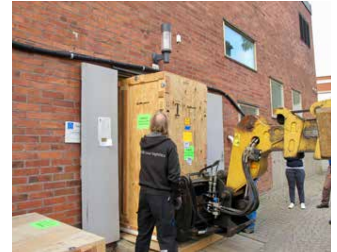
Above: The racks (in their protective crates) barely fit through the doorway to the entrance area of the PDC computer hall.
