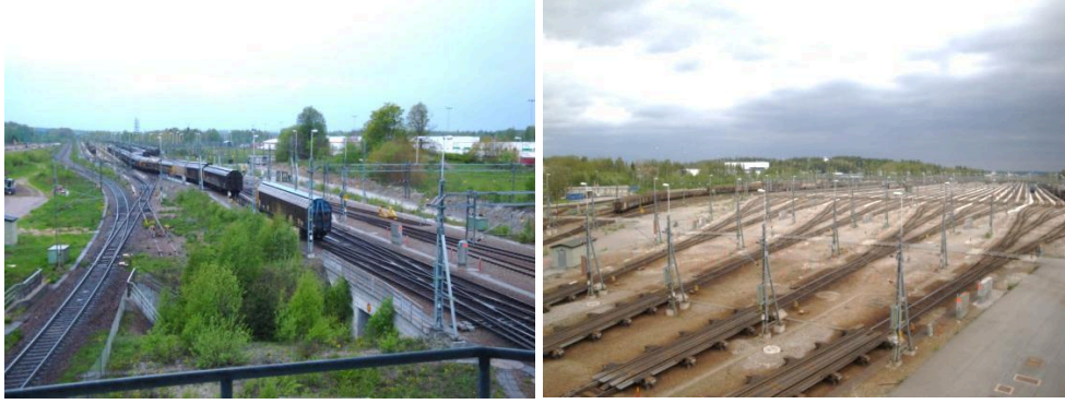
Figure 3: Hallsberg view from tower, Left: Hump, Right: Classification yard
