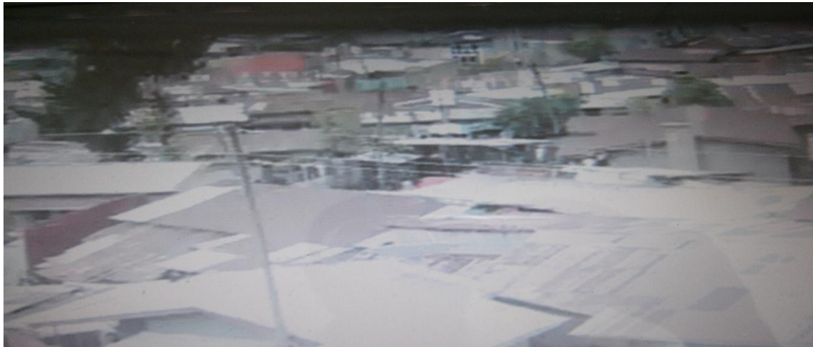
Photo 9-1: The Senga-Tera Redevelopment Locality before demolish
