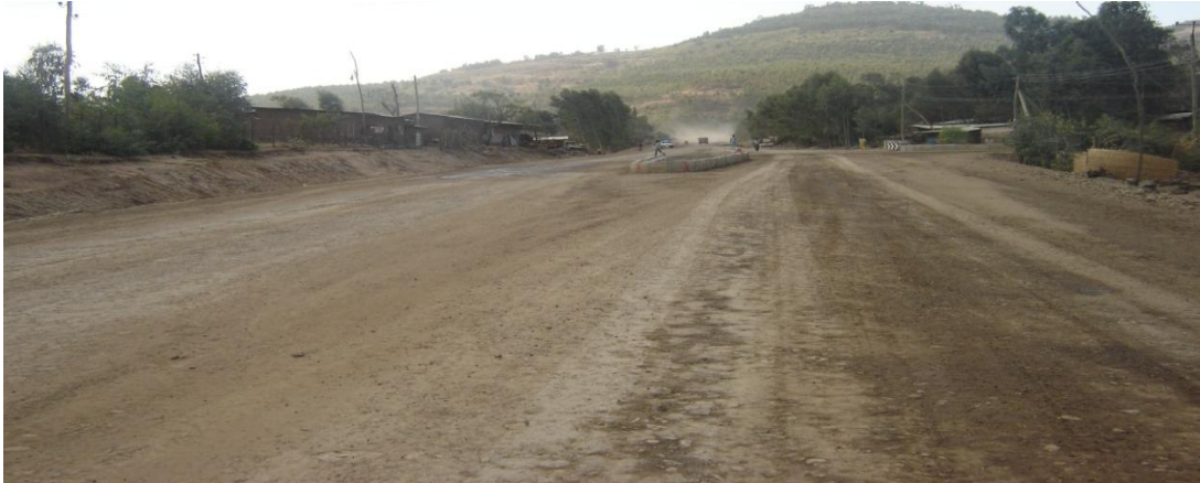
Photo 11-1: Gondar area of the Gondar-Debark Road redevelopment being under construction
