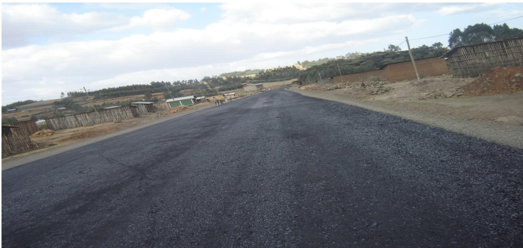
Photo 11-2: Wogera area of the Gondar-Debark Road redevelopment under construction
