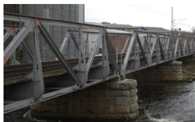
Figure 1. Lundamo railway bridge.
