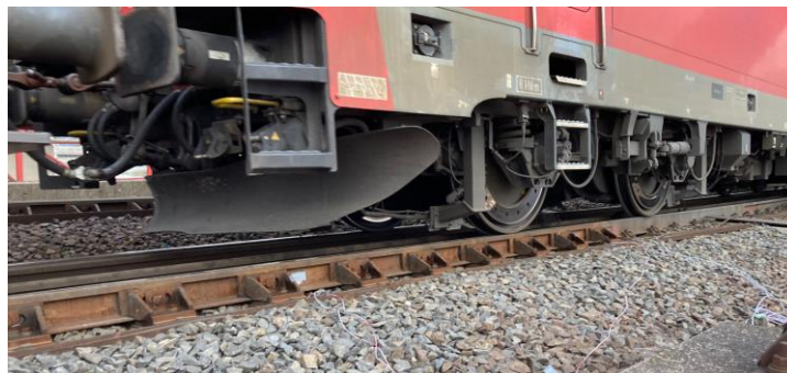
Figure 1. Field measurement directly on a rail expansion joint during a train crossing.
