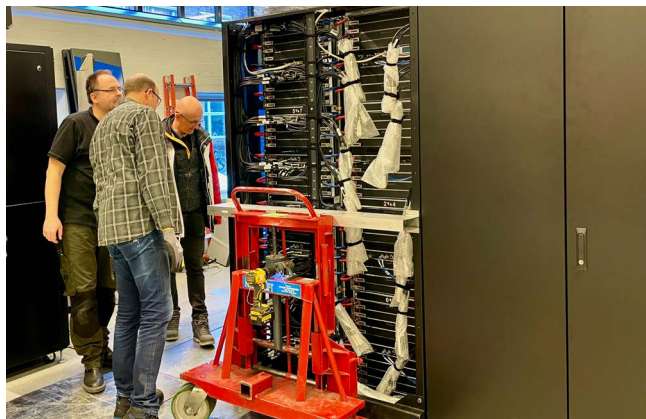
Below: The new CPU rack has just been moved into place.
